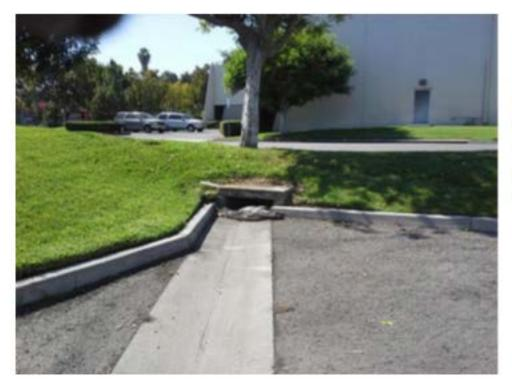
Obtain a stormwater sample as it falls into the storm drain (not from a puddle or stagnant water) <u>after</u> passing through the berm filters in front of the storm drain.
